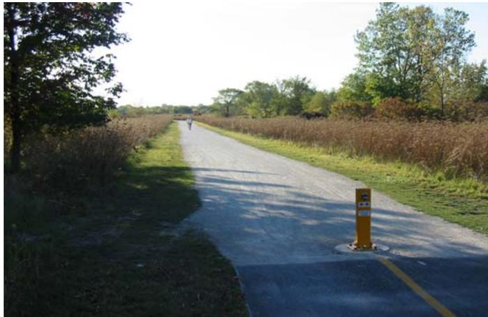
**Figure 5 – Trail Surfaced with Limestone Screenings**
